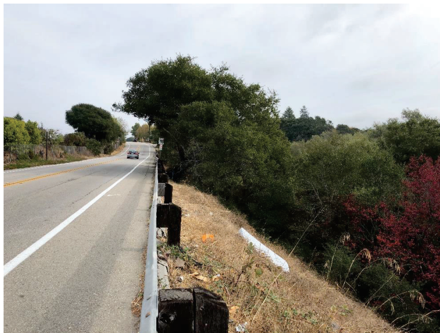
Photograph 5: Stormwater pipeline alignment along Soquel Avenue looking east toward Rodeo Creek Gulch (Source: Mori 2020).
