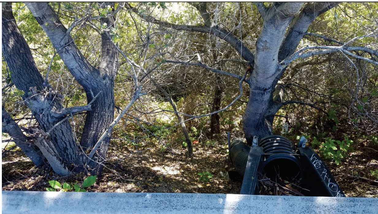
Photograph 10: Existing stormwater drain along Soquel Avenue looking south (Source: Ifland 2020).
